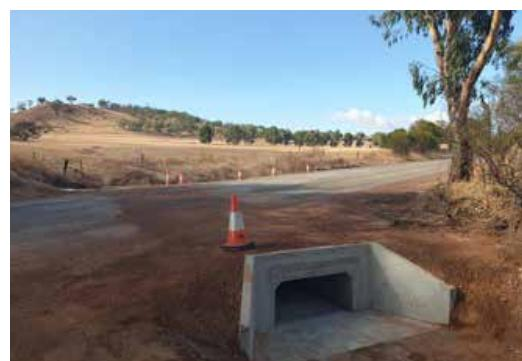
*Completed culvert crossing and headwall.*
