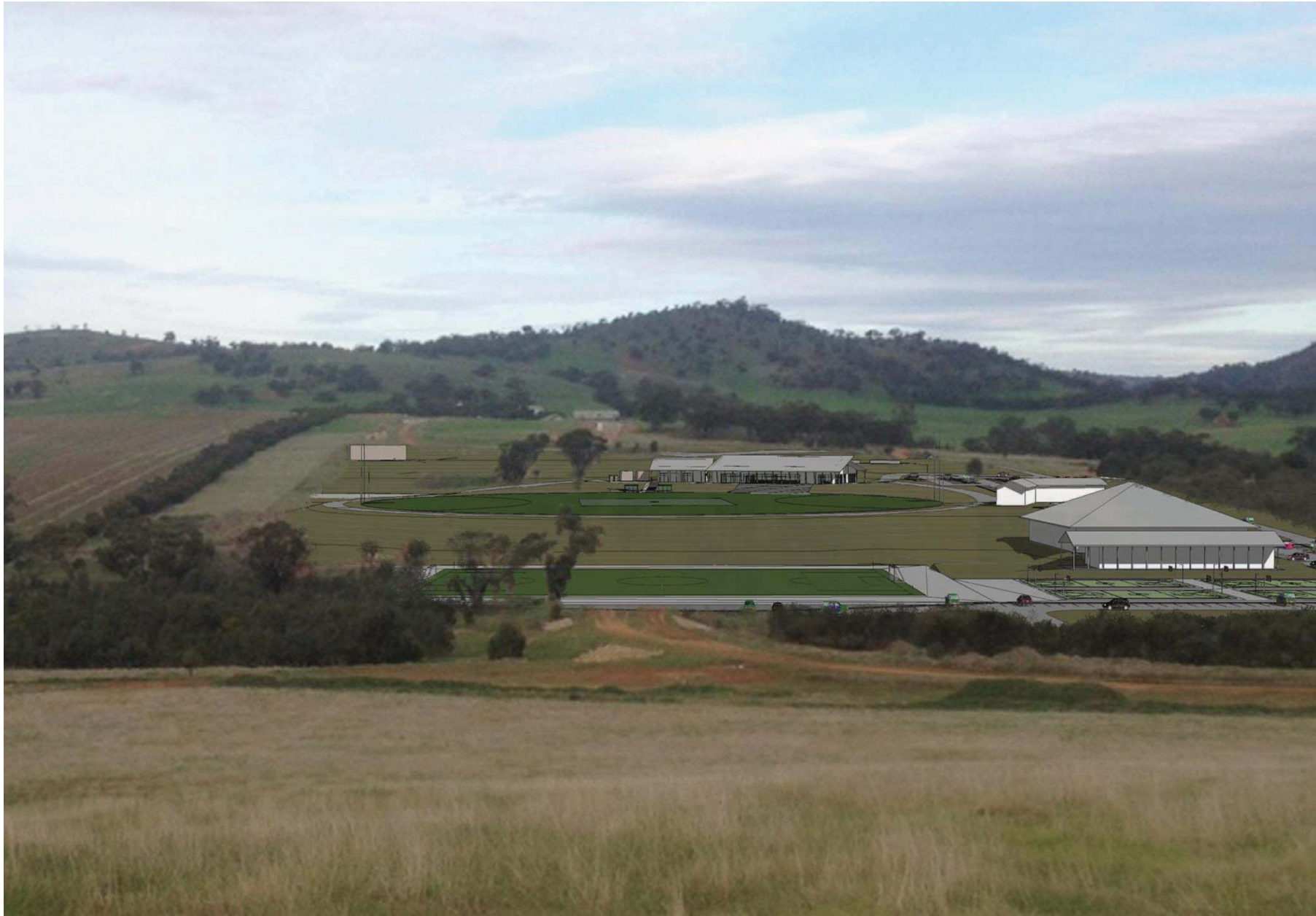
Toodyay Sport & Recreation Precinct - Site Photo ( After )
