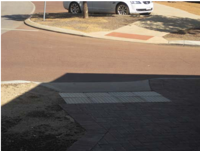
Charcoal Lane and Duke Street intersection showing pram ramp orientation directing path users to the middle of the intersection.
