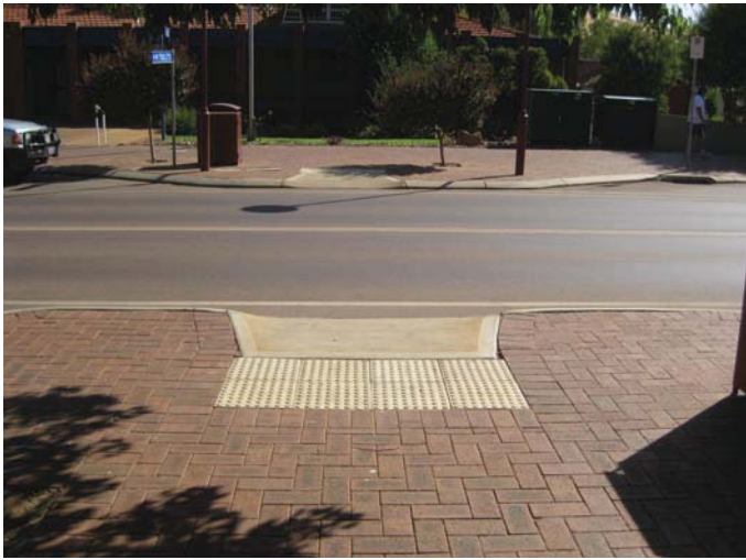
Stirling Terrace – showing typical construction of a pram ramp with tactile pavers set outside the actual ramp section.
