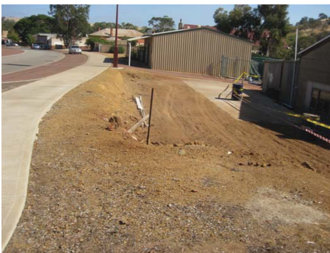
Charcoal Lane showing the steep batter in close proximity to the pathway adjacent to the laundry.
