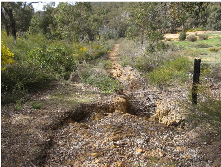
Figure 2. Damage to a firebreak from water run-off leaving the track impassable
