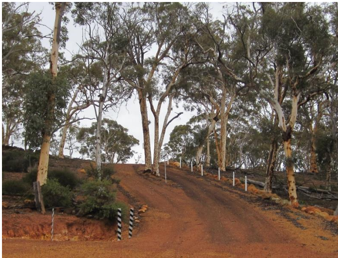
Figure 4. Tree located in the middle of Track 5F below a blind crest
