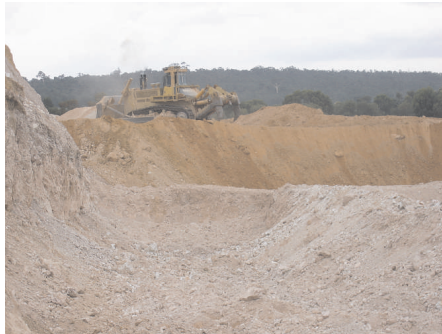
PHOTO 1 Bulldozer moving material
