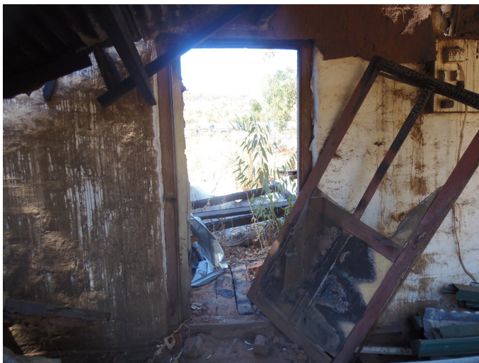
View of entry door from verandah.
