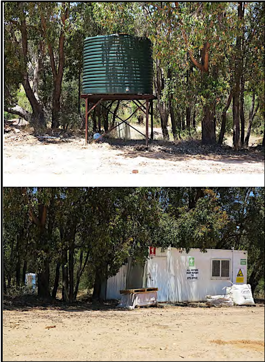
Figure 8 Non potable water supply tank above and site storage and serviced portable toilet below
