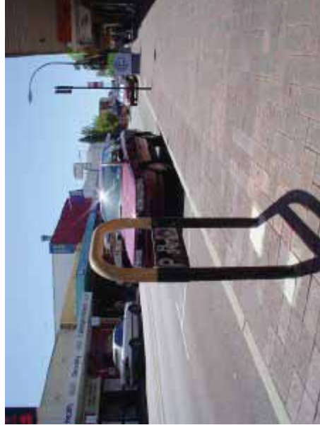
The standard bicycle parking U-rail – this example is on Albany Highway in East Victoria Park. There are numerous locations in Toodyay where parking rails should be installed.
