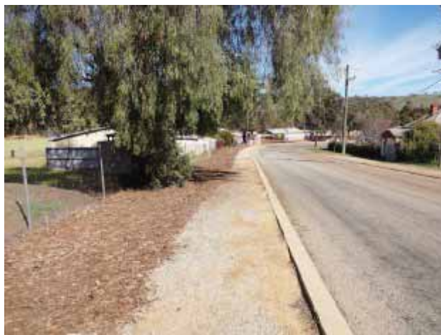
Construction of a shared path along Toodyay St, between Telegraph Rd and Jubilee St (to the Showgrounds) was recommended in the 2004 Bicycle Plan. It remains as one of projects yet to be implemented.
