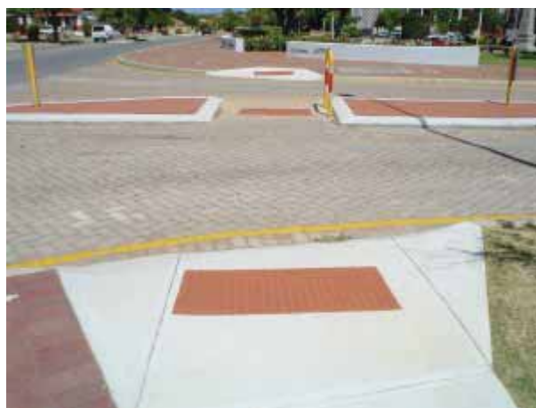
3-plane ramps, and tactile markings, are features of modern day, good quality road crossings. A similar standard crossing has already been used in the recently constructed paths and ramps in Toodyay.
