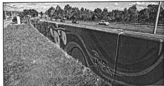
Public Transport Authority Project
