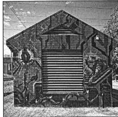
Public Transport Authority Project
