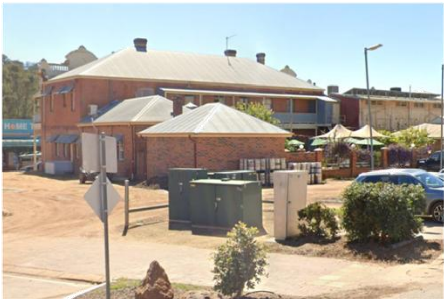
SIDE STREET VIEW SHOWING THE EXISTING REAR ALFRESCO AREA
