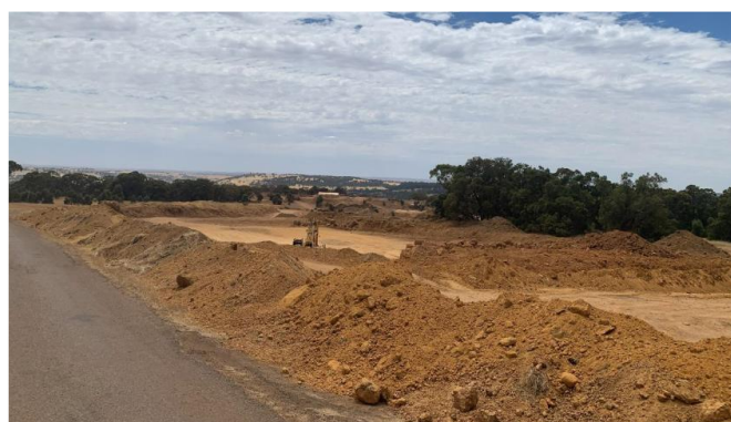
Picture 11.6.3: Example of Overburden to form perimeter bunds.
