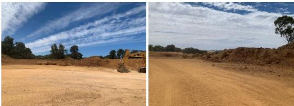
Current Excavation areas
