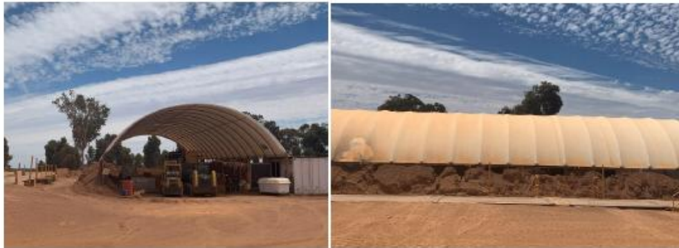
Dome shelter for vehicle maintenance
