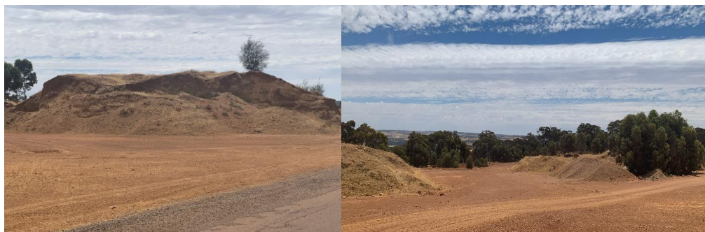
Pictures 11.6.2: Examples of Topsoil set aside for rehabilitation
