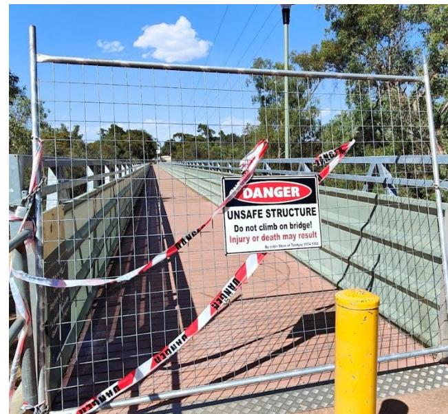
A full replacement of the decking is now required to ensure public safety and maintain the integrity of this critical piece of infrastructure.
