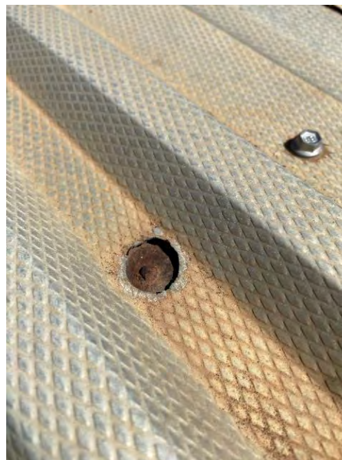
PICTURE 22 – GALVANIC CORROSION AT SCREW LOCATION.
