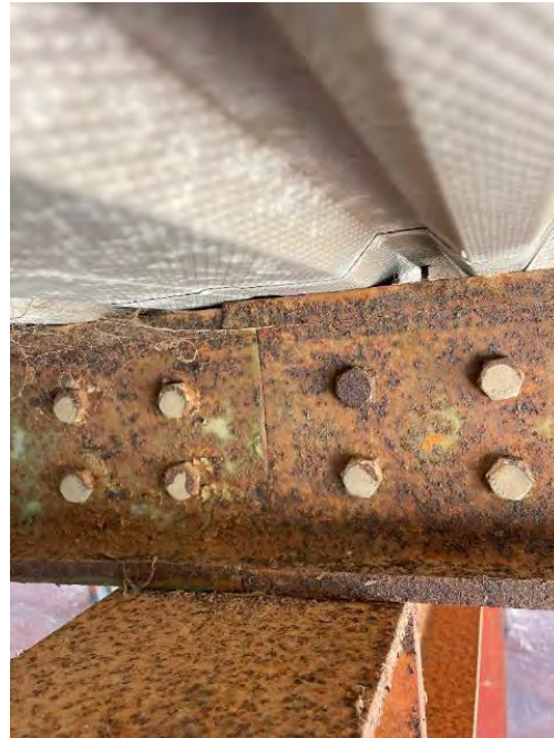
PICTURE 16– TYPICAL 'DOUBLED-UP' PURLIN CONNECTION
