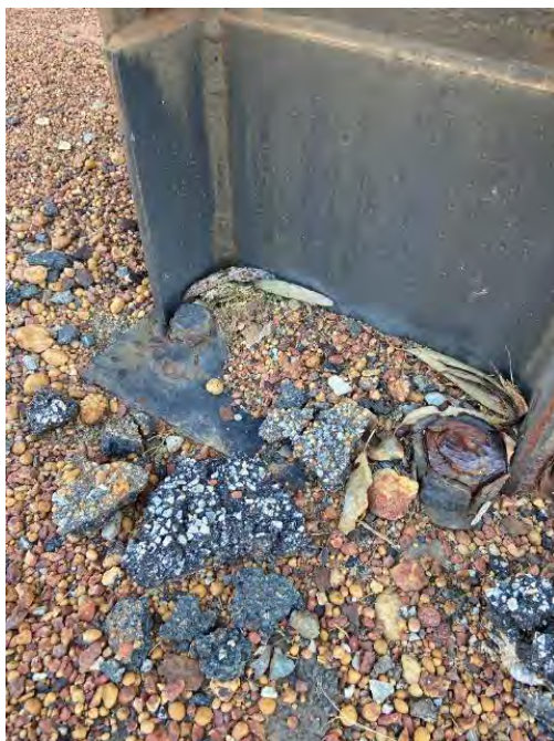
PICTURE 1 – CONCEALED BASE PLATE
