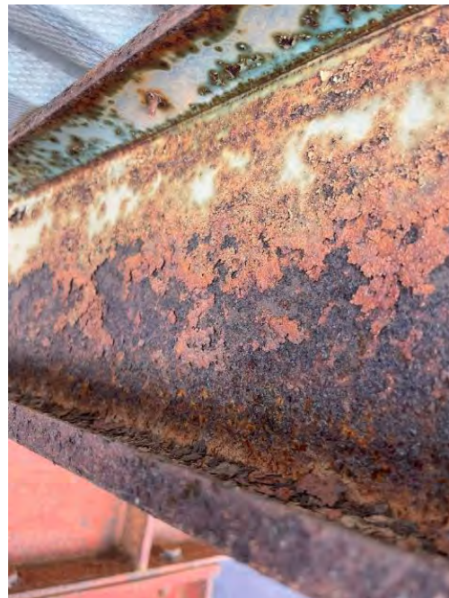
PICTURE 18 – TYPICAL PURLIN CORROSION EXAMPLE
