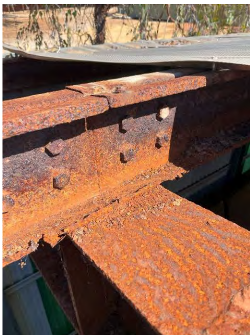
PICTURE 13 – SEVERE CORROSION TO PURLIN
