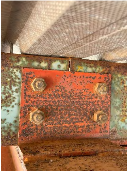
PICTURE 15 – TYPICAL PURLIN CLEATED CONNECTION
