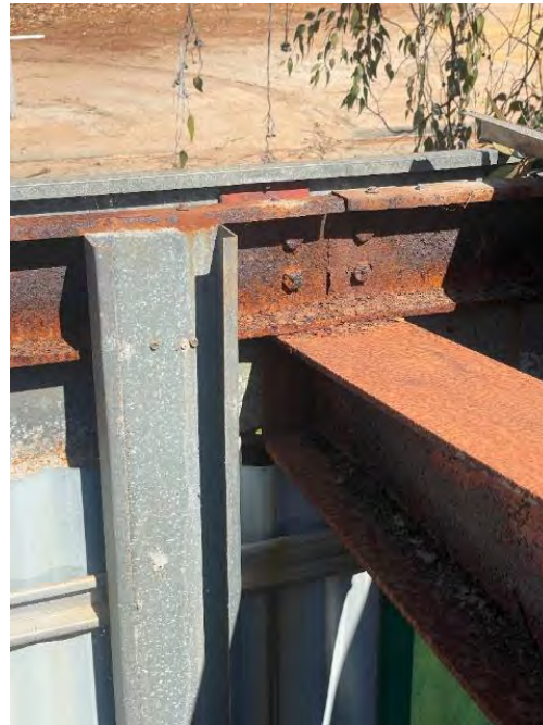
PICTURE 28 – COLUMN TOP CONNECTION
