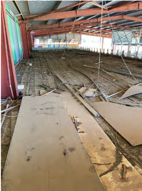
PICTURE 31 – COLLAPSED CEILING
