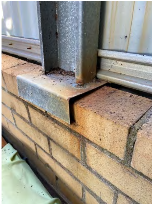
PICTURE 27 – COLUMN BASE CONNECTION
