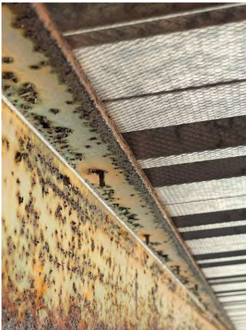
PICTURE 17 – TYPICAL PURLIN CORROSION EXAMPLE
