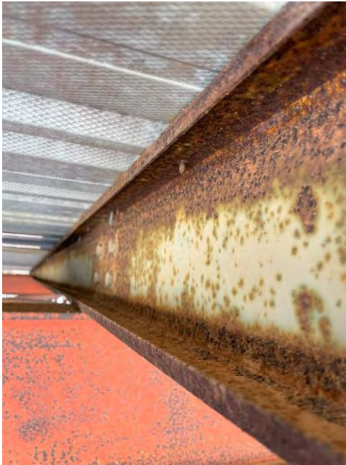
PICTURE 19 – TYPICAL PURLIN CORROSION EXAMPLE
