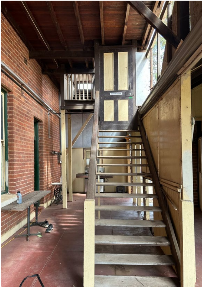
Image of the rear stair proposed to be removed.
