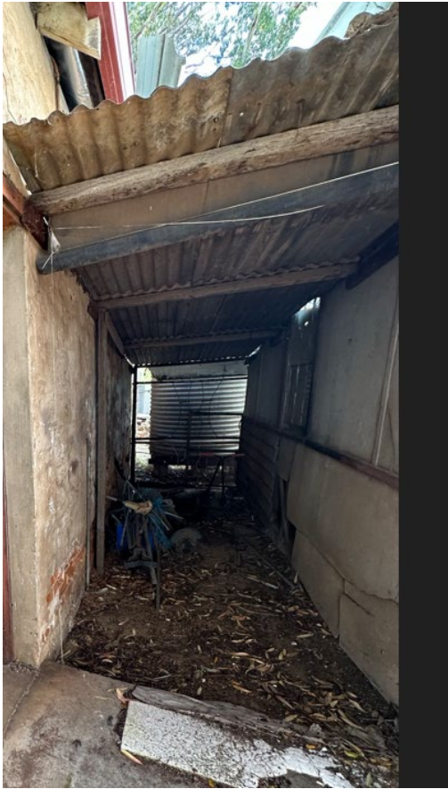
Boiler room to right of laundry
