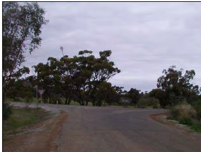
Figure 1 – View of Goomalling-Toodyay Road / Drummond Street East intersection looking South
