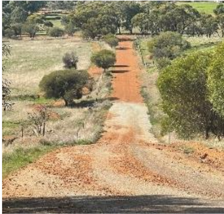
Photo 1- Emergency Access Way - Fawell Road - Church Gully Road (03/06/2022)
