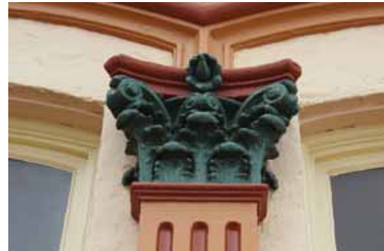
Ornate Victorian plasterwork detail
