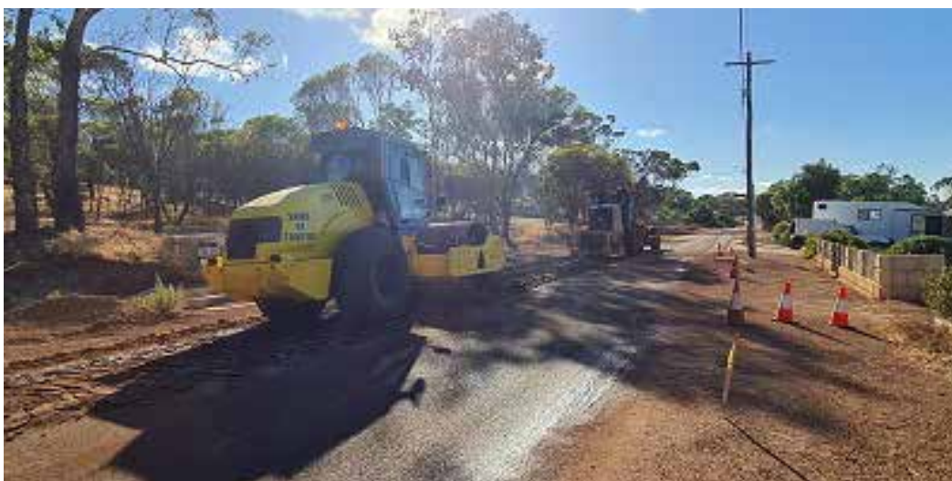
Toodyay Street upgrade – Ripping of existing asphalt
