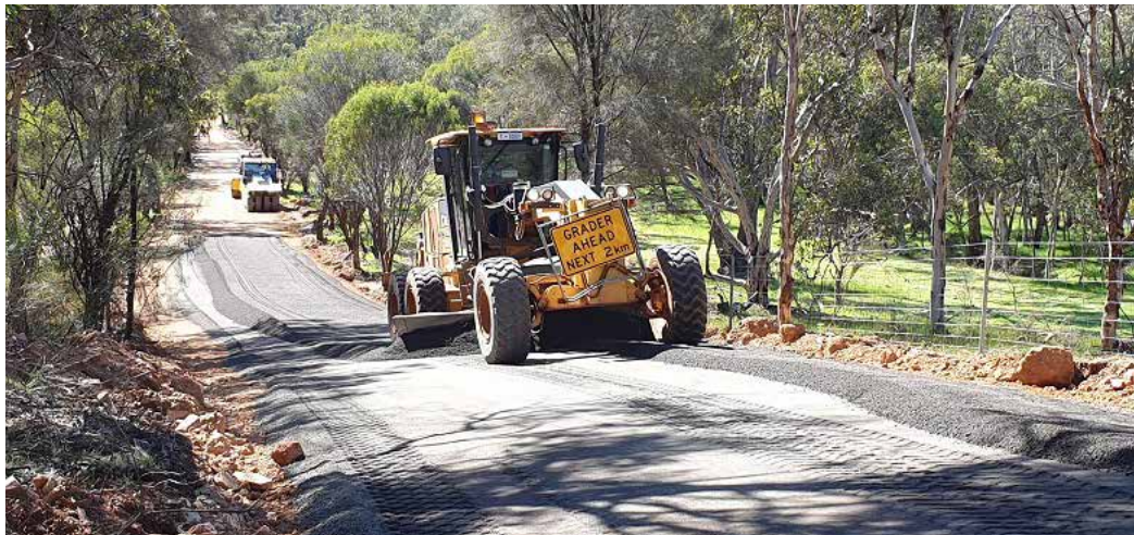
Morangup Road re-sheeting
