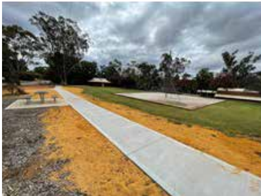
Duidgee Park – Completed footpath
