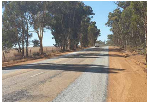
Completed shoulder widening and sealing
