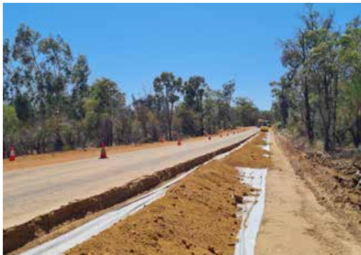
Toodyay Bindi-Bindi Road – Geotextile for soil stabilisation
