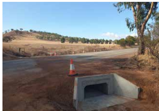
Completed culvert crossing and headwall.
