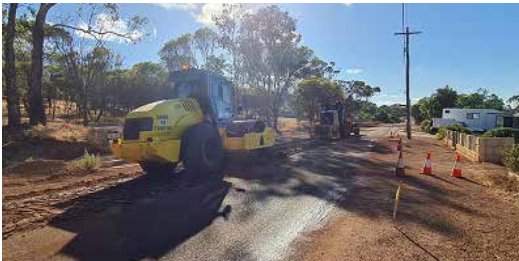
Toodyay Street upgrade – Ripping of existing asphalt
