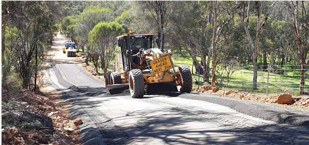
Morangup Road re-sheeting
