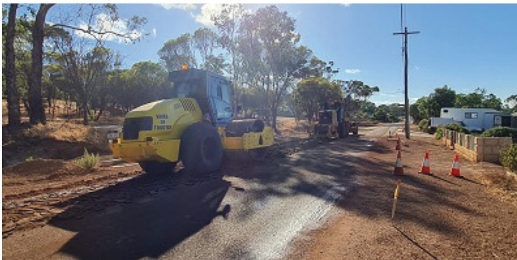
Toodyay Street upgrade – Ripping of existing asphalt
