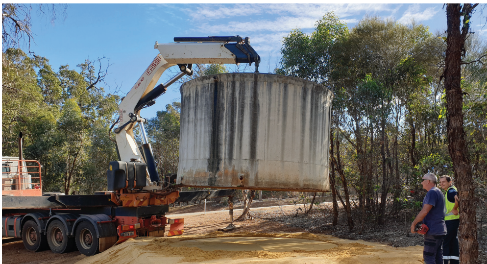
Relocating a fire emergency water tank from the decommissioned Coondle Fire Shed to Darwinia Road
