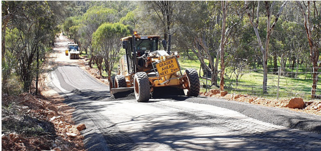
Morangup Road re-sheeting
