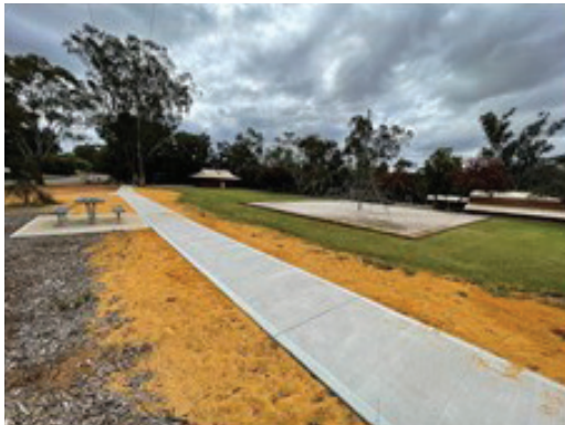
Duidgee Park – Completed footpath
