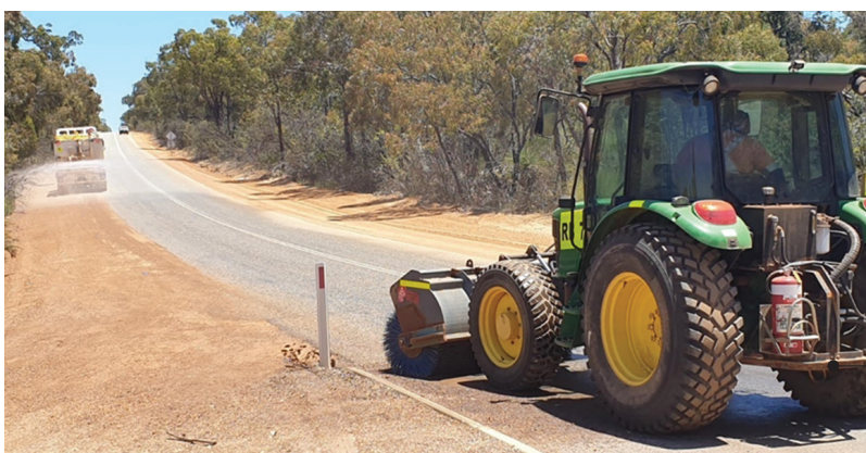
Edge break and shoulder works
