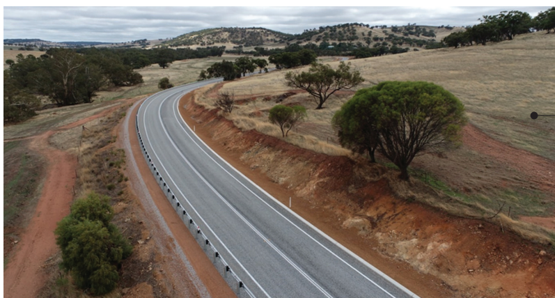
Bindi Bindi-Toodyay Road W-beam barrier rail and line marking
