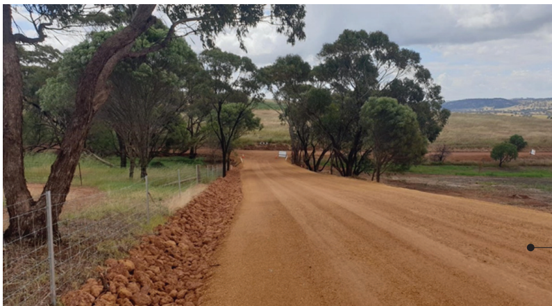
Re-sheet and rock pitching of open drain
