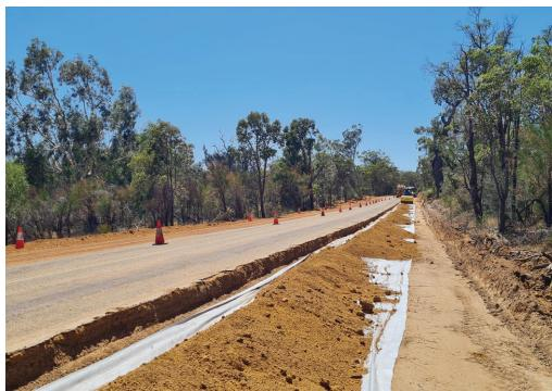
*Toodyay Bindi-Bindi Road – Geotextile for soil stabilisation*
