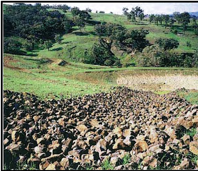
Figure C 6 Examples of rip rap and stone pitching to manage water on slopes, slow the water flows. All detention basins will be provided with rock pitching to protect the outlets
