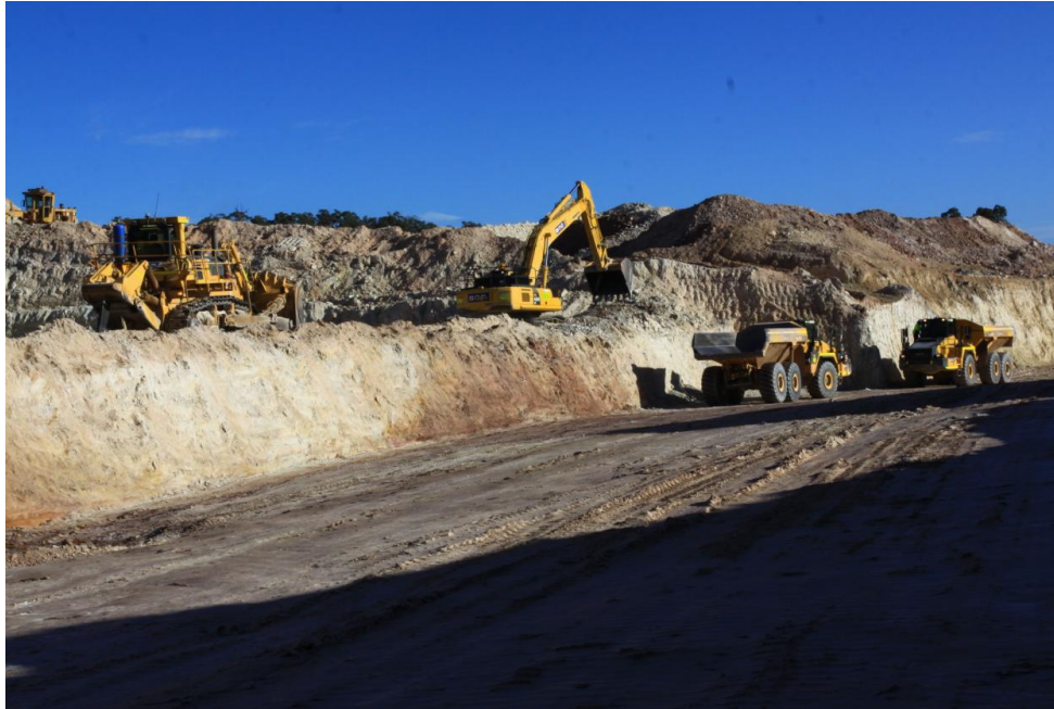
Photo 5. Loading with excavator into dump trucks.
