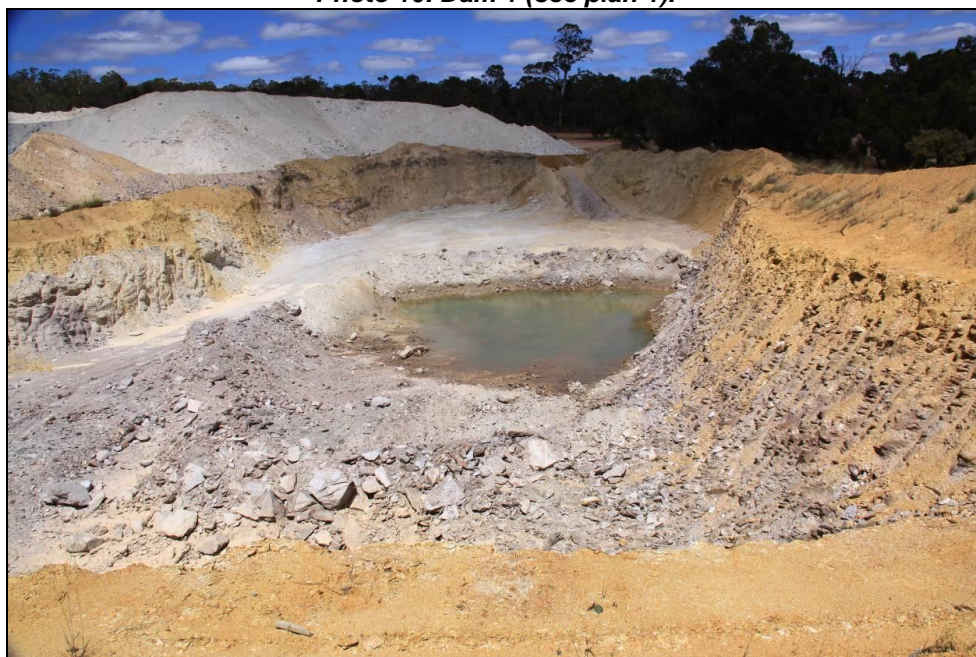
Photo 11. Dam 2 to retain stockpile runoff.
