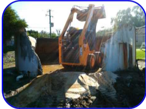
Removal of old showground water tank
