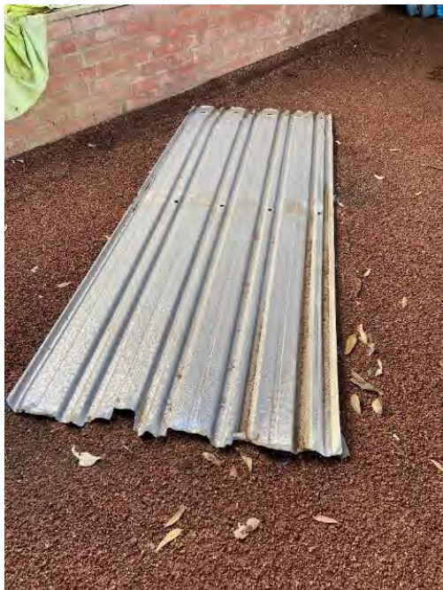
PICTURE 21 – ALUMINIUM ROOF SHET PROFILE
