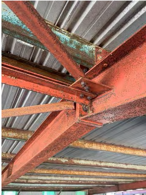
PICTURE 9 - TYPICAL RIDGE/BRACING/STRUT CONNECTION
