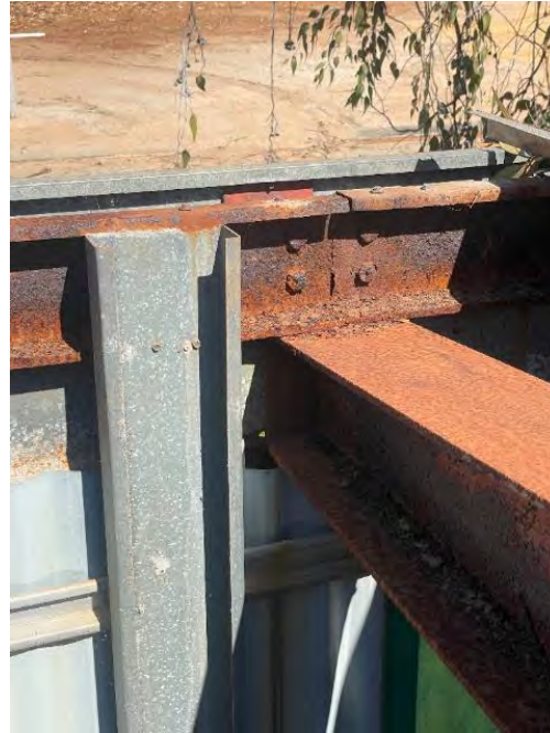
PICTURE 28 – COLUMN TOP CONNECTION
