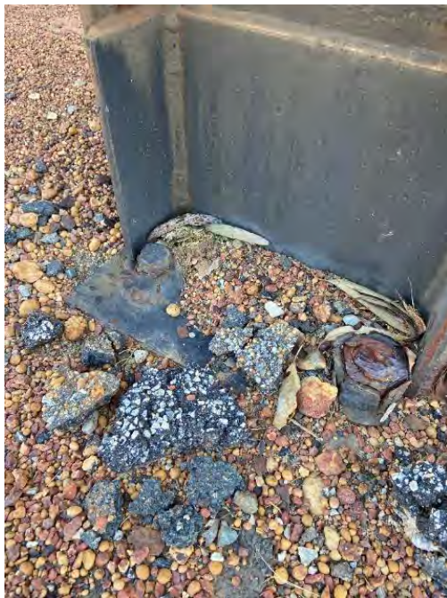
PICTURE 1 – CONCEALED BASE PLATE
