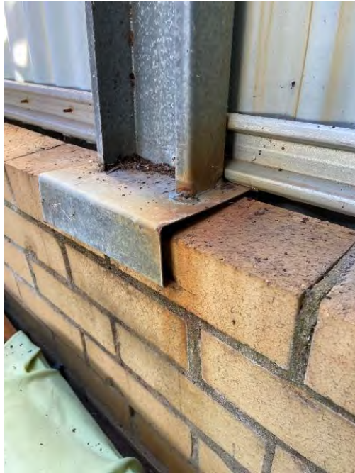
PICTURE 27 – COLUMN BASE CONNECTION
