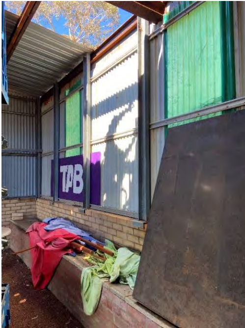
PICTURE 29 - TYPICAL ENCLOSED SIDE OF STRUCTURE
