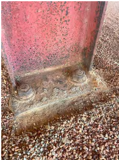
PICTURE 5 – BASE PLATE CONDITION INTERNAL & PROTECTED FROM WEATHER
