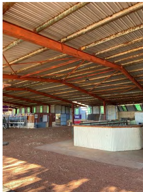
PICTURE 8 – TYPICAL STEELWORK LAYOUT
